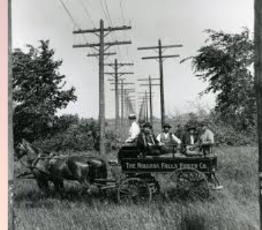
TRANSMISSION LINES 1902 NAYAGRA POWER CORPORATION(11KV)
